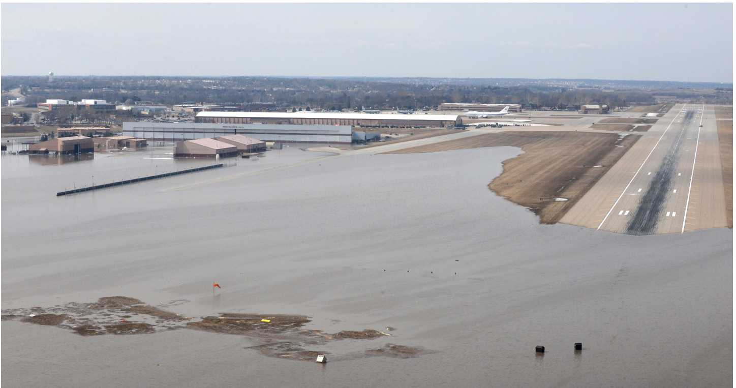
March 2019 flooding at Offutt Air Force Base, Nebraska, limited runway use, even after floodwaters receded, due to inspection requirements. The new STRATCOM headquarters building, completed earlier in 2019, was built on higher ground, with barriers to reduce flood risk, and thus was not affected by the flooding. (Department of Air Force photo by Tech Sgt Rachelle Blake)
