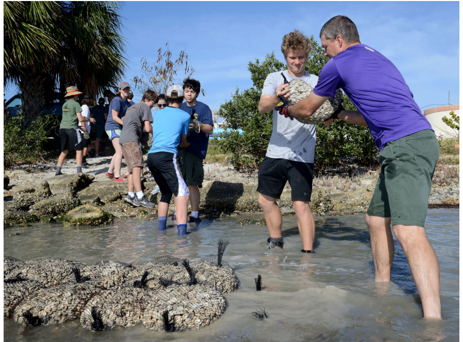
Members of MacDill Air Force Base and the local community build oyster reefs at MacDill Air Force Base, Florida, March 30, 2018. MacDill's eastern shoreline is prone to erosion, however oyster reefs aid in stabilizing the shoreline as well as improving MacDill's vast natural habitats. This build is part of the ongoing Oyster Reef Shoreline Stabilization project, which started in 2004. (Department of the Air Force photo by Staff Sgt Tori Long)
